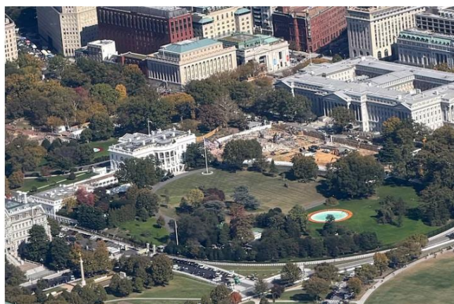
Figure 11 – Aerial photograph of President’s Park and the surrounding area on October 23, 2025. The site of the former East Wing is to the right of the remainder of the White House. ABC News / Katie Harbath.
