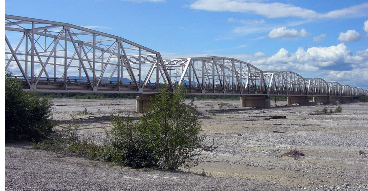
Gerstle River Bridge, AK
