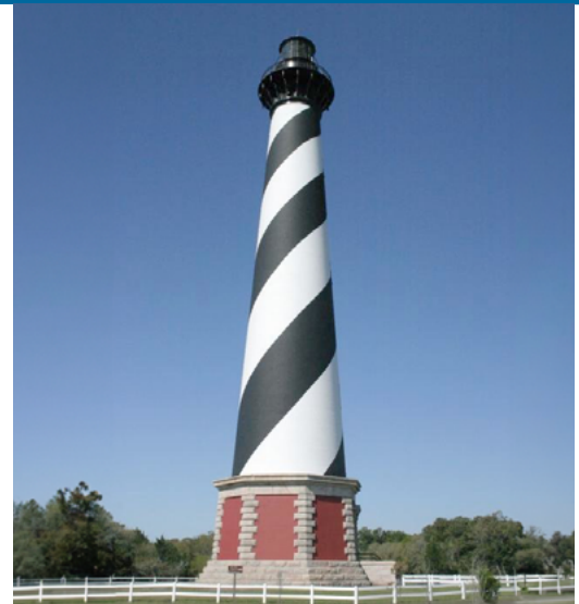
National Park Service-funded projects to repair deferred maintenance and preserve historic sites include the Cape Hatteras Lighthouse Restoration Project. Designed in the late 1800’s, this National Historic Landmark in North Carolina is the tallest traditional lighthouse in the United States.
